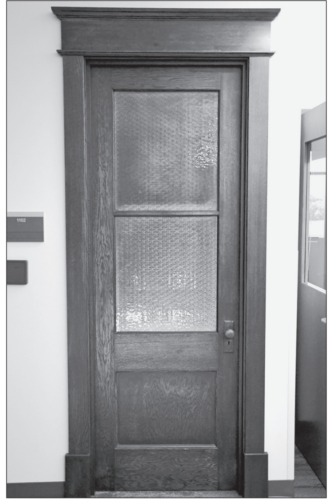
Design elements for the new Justice Center include the use of the door from the old sheriff's office into the new sheriff's office.
